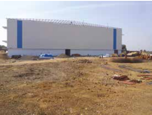
USED IN WAREHOUSE
