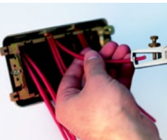
Fit installation box and mounting grid. Pull through cables, cut and strip to length.
