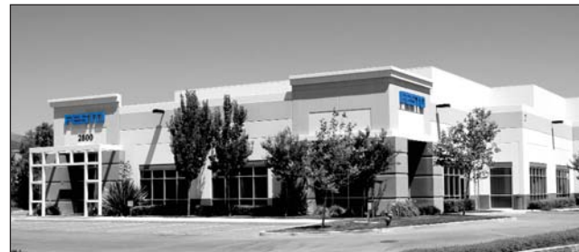
West: 2800 Collier Canyon Road, Livermore, CA 94550
